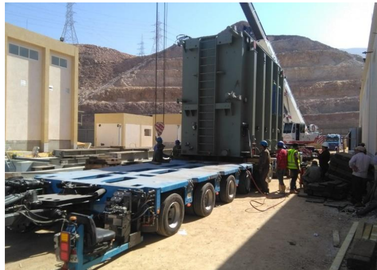
Discharging, Trucking & Unloading to foundation for 2 Siemens Transformers of 135 tons each from Alexandria port to El Galala City.
