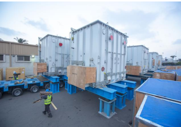
Offloading and delivering 8 transformers each of 228Ton to the yard in Dekhila port
