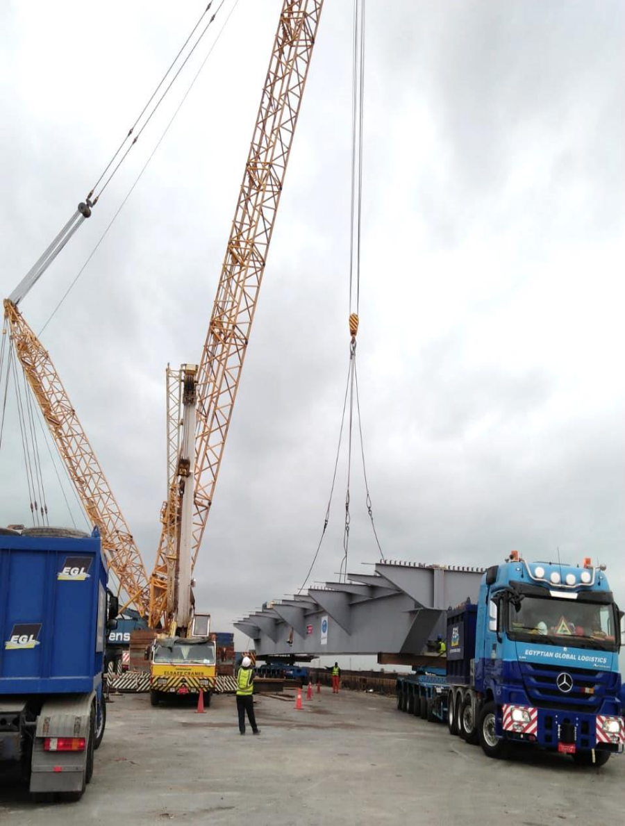
Transportation of 115 tons & 47 m long of Steel Structure for major Banha bridge.
