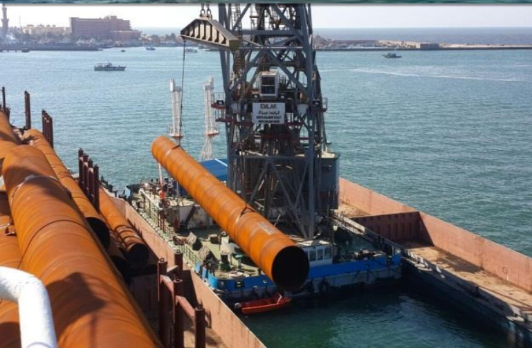
Discharging using floating cranes, Barging & transport of 47 tons 43 m steel pipes to the site at Port Said east new jetty.
